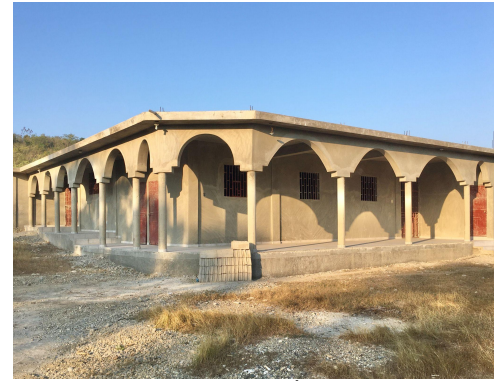
Current progress on clinic construction
